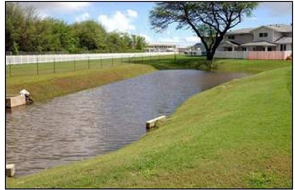
This photo, taken shortly after Charlotte Schaefer's drowning in February 2004 at Pearl City Peninsula, shows the drainage ditch and retention pond. Since the drowning, the Navy installed a safety barrier.
